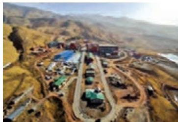
Gold processing plant
